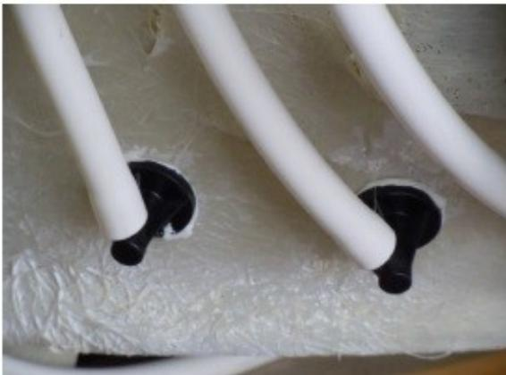
Real Air jets, not holes drilled in tub.
